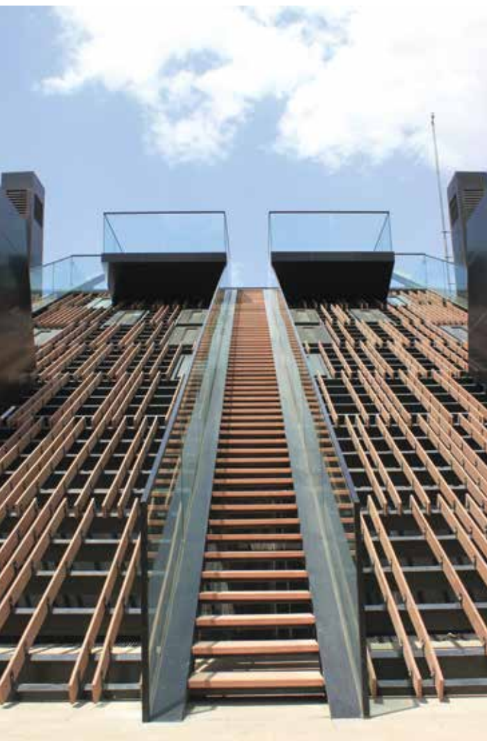
1) The slanting façade with a seven meter depth forms the identity of the building
